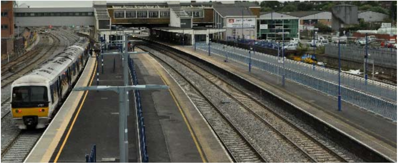
Banbury station after the changes. Note the former bay platform on the left now made wider and into a through road with a Chiltern unit awaiting departure.
